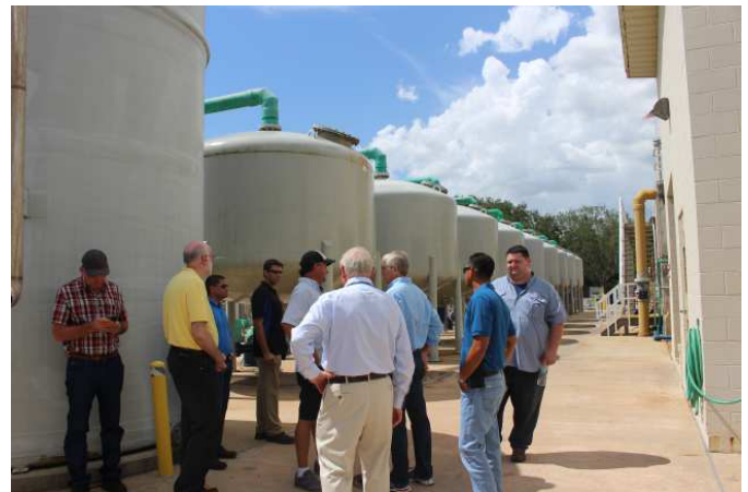
Some of the plant's many pressure filters.
