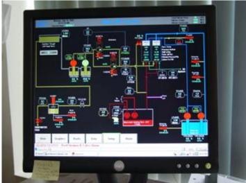
At the WTP, instrumentation and control upgrades for Stage 1 were provided primarily by Pall Corporation in the form of a main A-B ControlLogix PLC and remote drops for each filter rack and CIP system. Pall Corporation also provided the main operator HMI station in the WTP office, remote programming modem, and Ethernet router. This allowed the WTP to monitor the new pump house PLC and for Pall to have the ability to provide remote troubleshooting and programming upgrade services.
