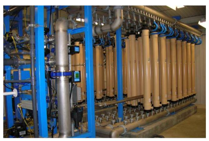
The WTP upgrade became a two stage, multi-year project spanning from 2002 to 2009. Stage 1 involved baffling the adjacent potable water reservoir and construction of a new distribution pump house to take advantage of the new baffling arrangement. In addition, Pall Corporation Microza<sup>TM</sup> MF pressure membranes were installed in parallel with the existing conventional treatment process, providing the redundancy required for the Stage 2 upgrades to proceed.
