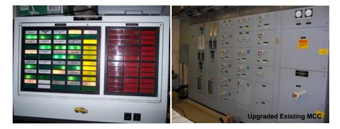
A Stage 3 had been planned whereby the river water intake pump house PLC would be upgraded to match the WTP PLCs once Stage 2 was completed. This upgrade was moved ahead and added into Stage 2 and consisted of replacing an obsolete GE PLC with A-B ControlLogix with a local control panel touch screen HMI communicating back to the WTP via Ethernet using an existing direct buried multi-pair instrument cable.
