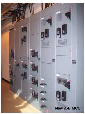
and breakers. All of the new electrical and control equipment were all networked together using DeviceNet resulting in reduced installation material, labor, and commissioning time.
