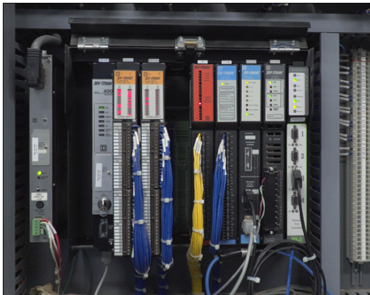
Figure 1- Old – end-of-life non-redundant controller
