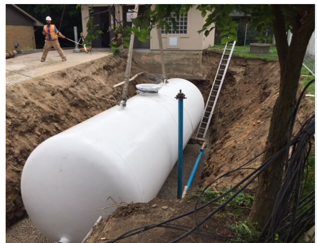
Figure 2 – Installation of the underground contact chamber
